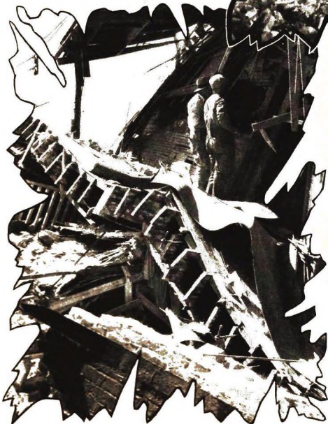
The Southern California quake of 1933 ripped away the walls of buildings in Long Beach, exposing living quarters to the gaze of everyone. Left: Here's what a good trembler does to a house.
